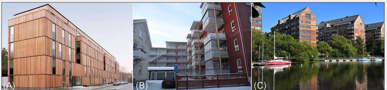
Fig. 8 - Examples of construction with modular systems in Sweden: (A) “Skagershuset”, prefabricated modules from the company Moelven built in 2013; (B) “Ekorren”, building system with glulam from the company Setra built in 2010; (C) “Strandparken”, CLT construction from the company Martinsons built during 2012-2017.
