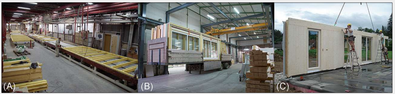
Fig. 7 - Examples of off-site prefabrication: (A) assembly of wall elements where the openings are constructed in a horizontal position; (B) wall elements on their way from the factory to the building site; and (C) assembly of modules. A building process with prefabricated components or modules is faster, less weather-sensitive and provides a better control over the costs.
