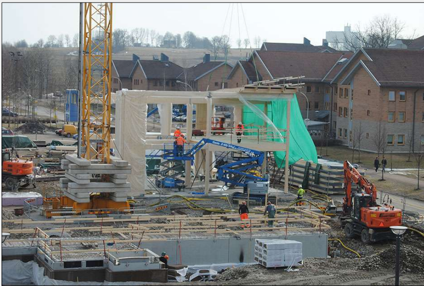
Fig. 5 - Glulam framework under erection for an educational building: “House N” at Linnaeus University in Växjö, Sweden (built in 2011).
