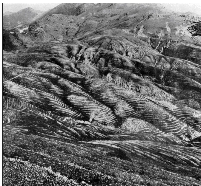
Fig. 7 - Soil preparation work for terraced hillslopes of Coscile basin (by CASMEZ 1964).
