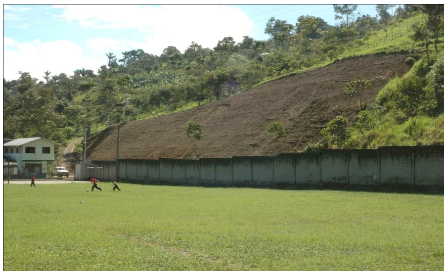
Fig. 2 - Live palisade following construction.
