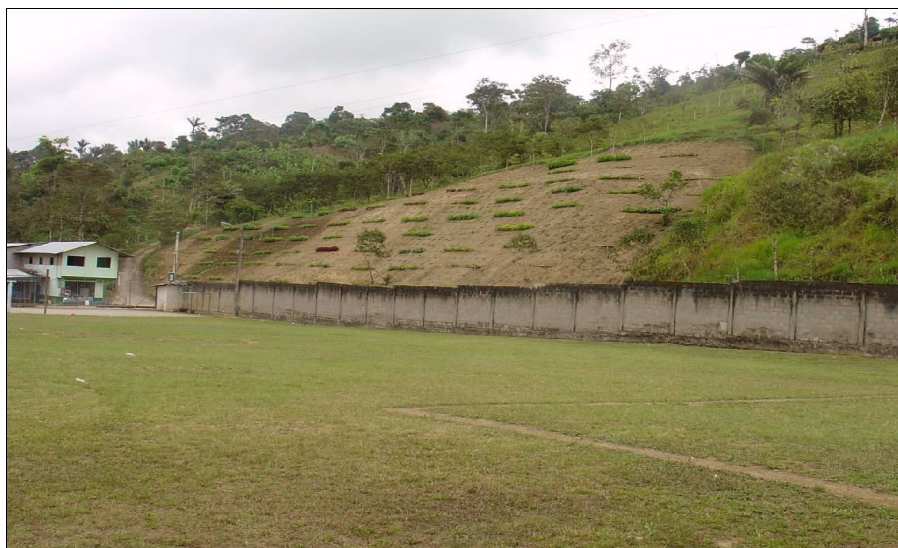
Fig. 3 - Live palisade two months following construction.
