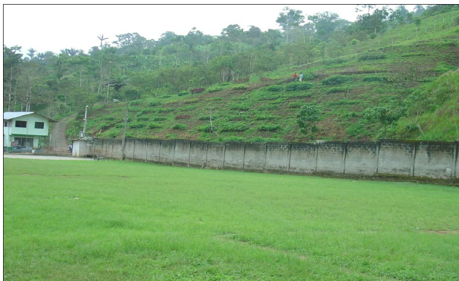
Fig. 4 - Live palisade five months following construction.
