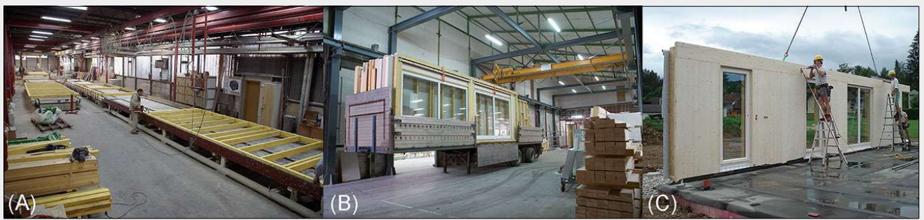
Fig. 7 - Examples of off-site prefabrication: (A) assembly of wall elements where the openings are constructed in a horizontal position; (B) wall elements on their way from the factory to the building site; and (C) assembly of modules. A building process with prefabricated components or modules is faster, less weather-sensitive and provides a better control over the costs.
