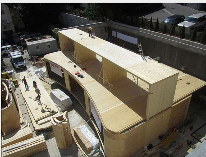
Fig. 6 - Prefabricated CLT elements are transported to the construction site and then assembled and erected manually: Waldorf School in Ljubljana, Slovenia built during 2009-2012.
