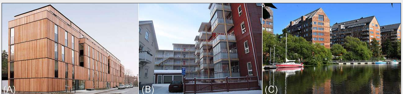
Fig. 8 - Examples of construction with modular systems in Sweden: (A) “Skagershuset”, prefabricated modules from the company Moelven built in 2013; (B) “Ekorren”, building system with glulam from the company Setra built in 2010; (C) “Strandparken”, CLT construction from the company Martinsons built during 2012-2017.
